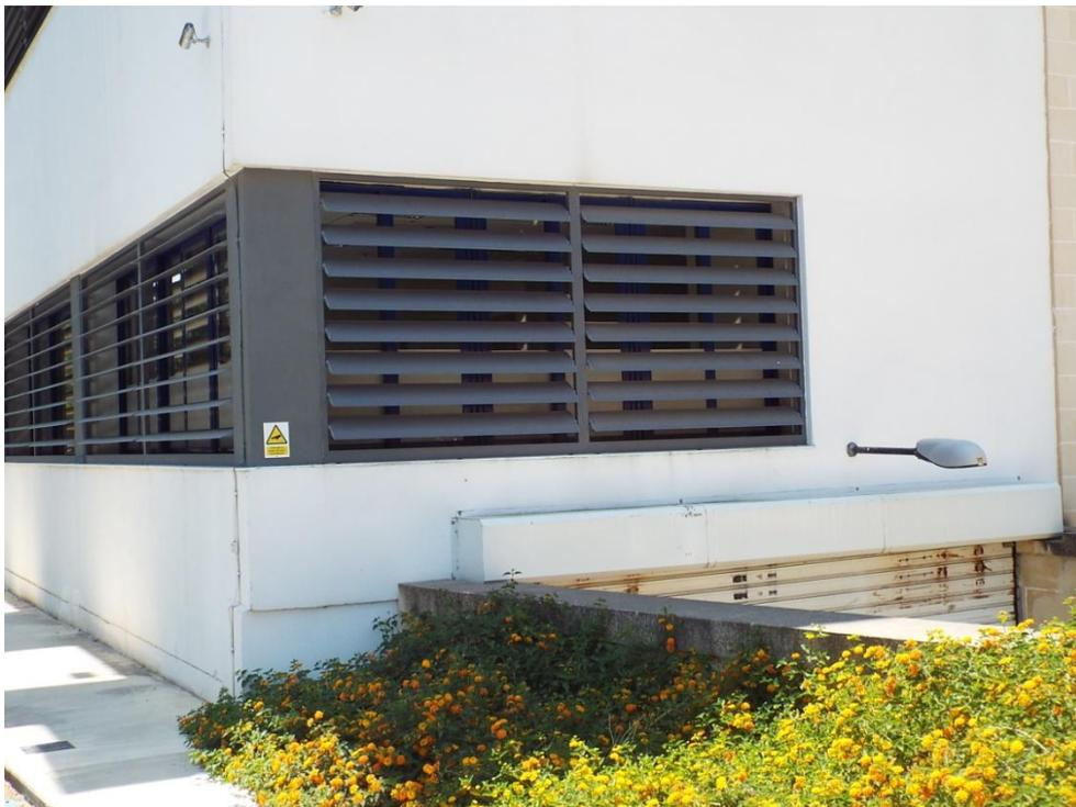
**Figure 2 External shading helps the spaces remain cooler by keeping sun's rays from entering inside. For windows and doors facing south the best solution is having horizontal shading over the windows (Refer figure 3). This may be part of the structure (ex. concrete) or made of lightweight materials**
