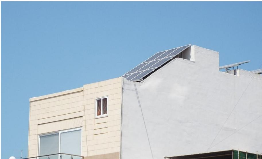
**Figure 5 Photovoltaic Solar panels integrated within the building**
